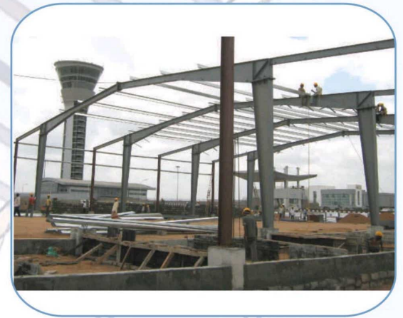
CIVIL WORK ON SITE
